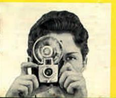
The picture shows the recommended way to hold the camera. It's important that you get a firm grip on the camera and that your finger or the neck strap is not in front of the taking lens. BATTERY BASE UP
